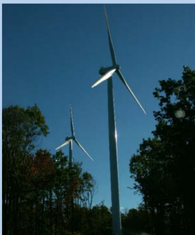
Wind turbines atop an Appalachian Mountain Ridge. USFWS photo
