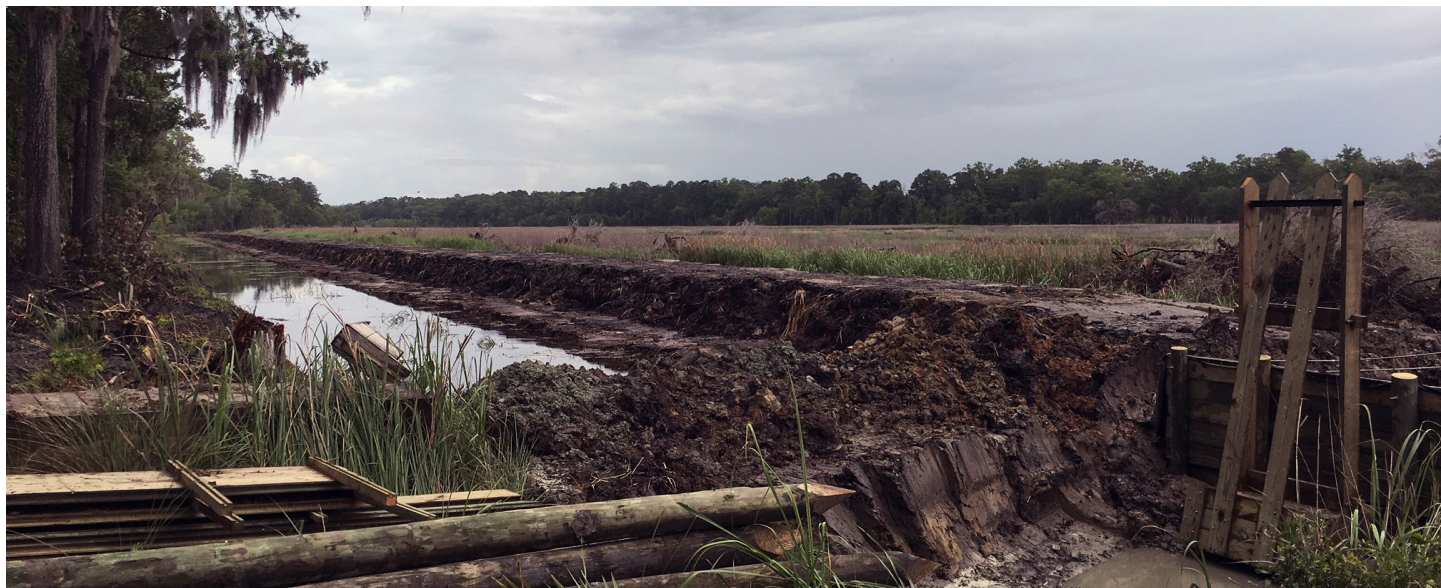
An example of management techniques for Black Rail: Installation of rice trunk and canals to manage water levels, and construction of dikes. Jason Ayers
