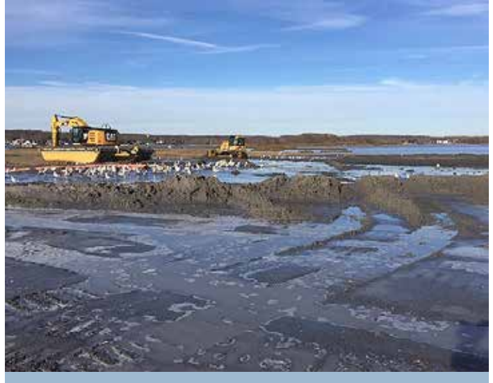
Low-pressure equipment, specially designed for work on soft ground like marshes and wetlands, was used to carefully place dredged soil on top of a marsh in Rhode Island. NOAA
