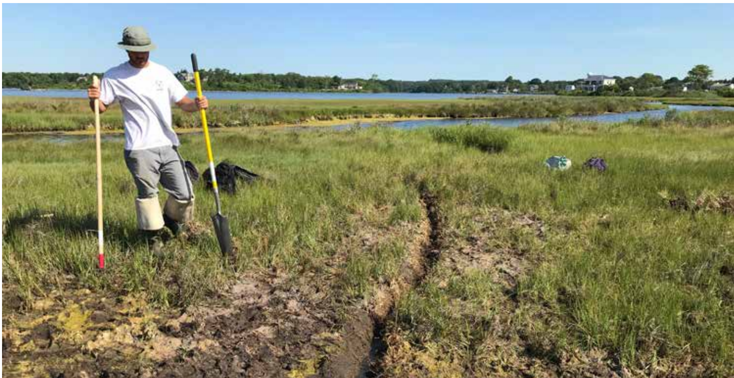
Creating shallow channels, or “runnels,” can reduce ponding and help restore natural hydrology in marsh systems with impaired drainage. Tanner Steves
