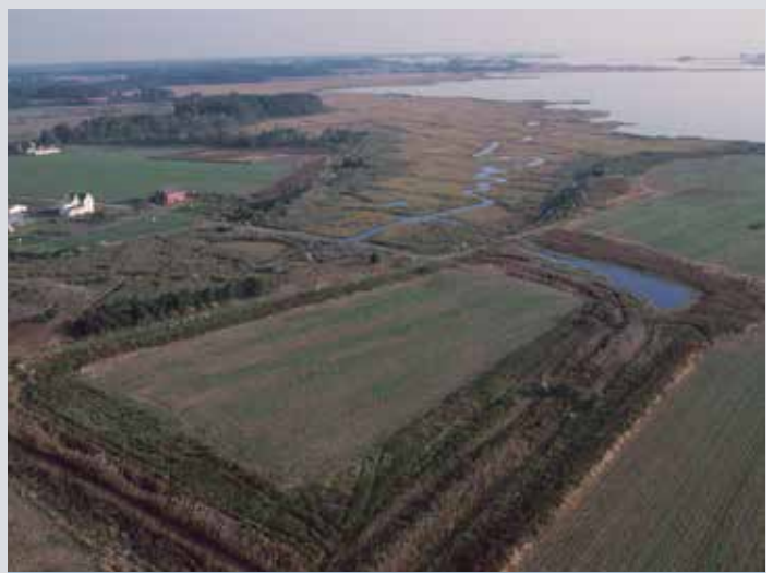
Low lying agricultural fields such as this one, in Wicomico County, Maryland, can suffer from saltwater intrusion. By grading and creating channels, the lowest portions can be restored to tidal wetlands, which improves the resilience and productivity of higher portions. Tim McCabe/USDA NRCS
