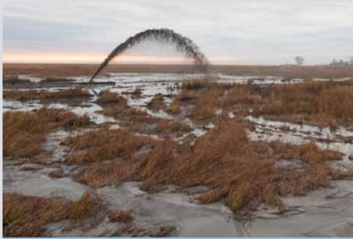
Thin layer deposition helps to raise marsh elevation and mitigate impacts of sea level rise. Dave Harp
